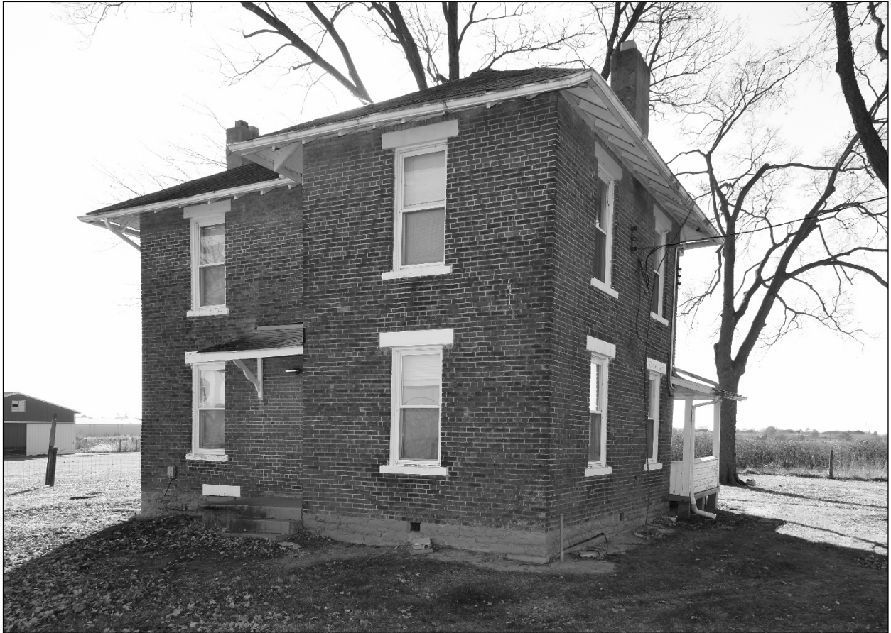
1. Northwest corner with front entry under the porch roof at left
