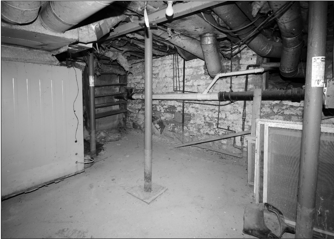
8. Basement looking southeast
