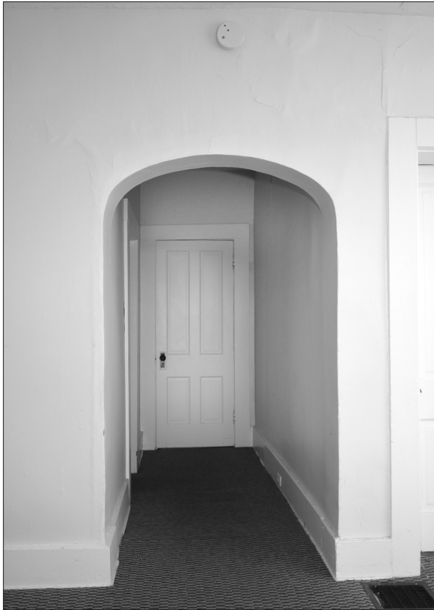
15. Arched opening on north wall of dining room to modern corridor created to access bathroom at left
