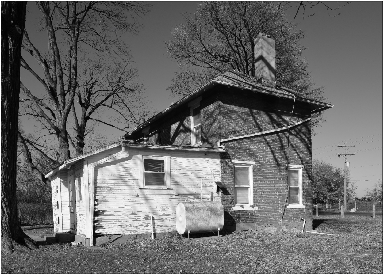
3. Southeast corner showing kitchen addition at left
