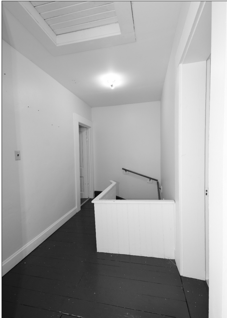
18. Second floor hall looking south
