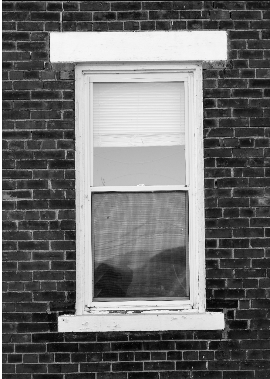
7. Detail of window on north elevation
