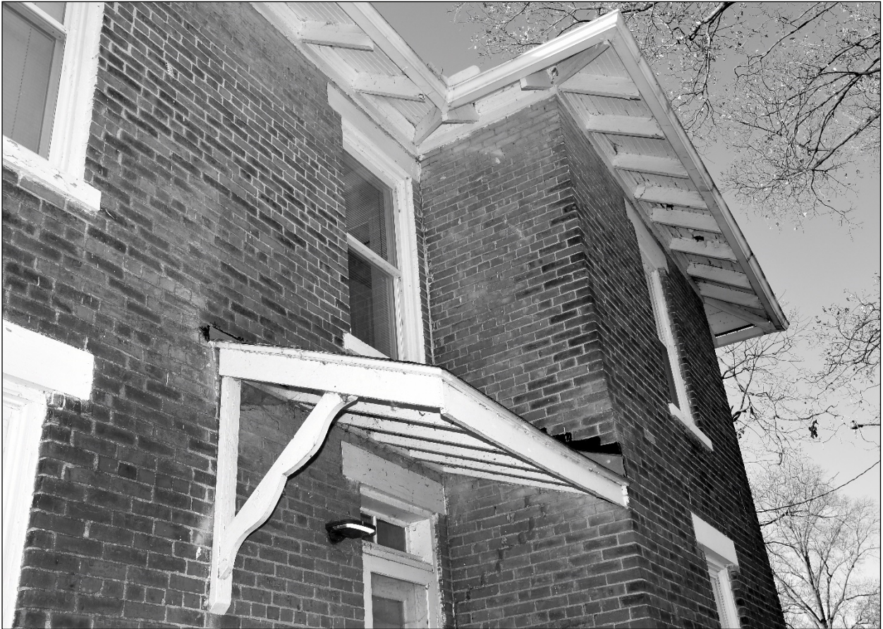
6. Detail of roof eaves along north elevation
